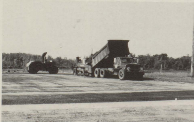
Tennis Court Construction
